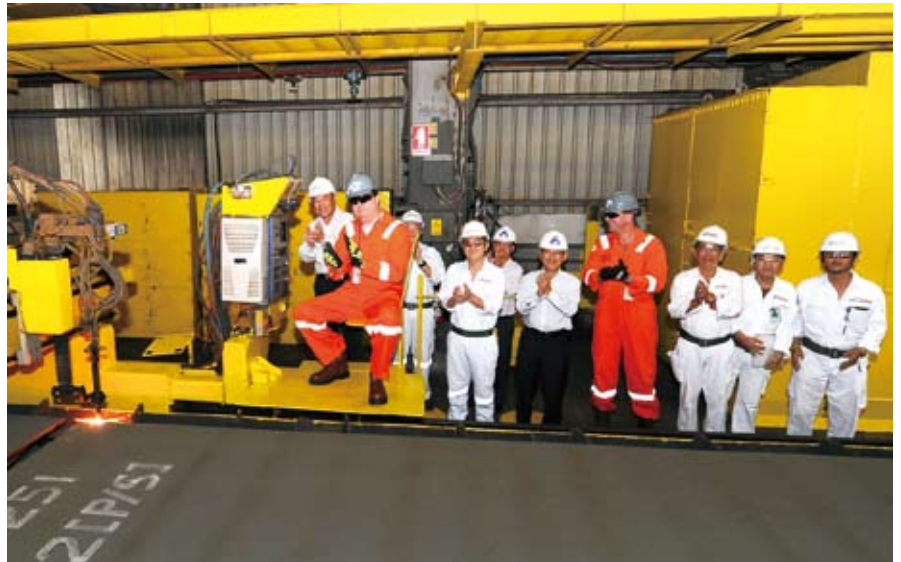
The first of Ensco's new series of KFELS Super A jack-up rigs strikes steel
